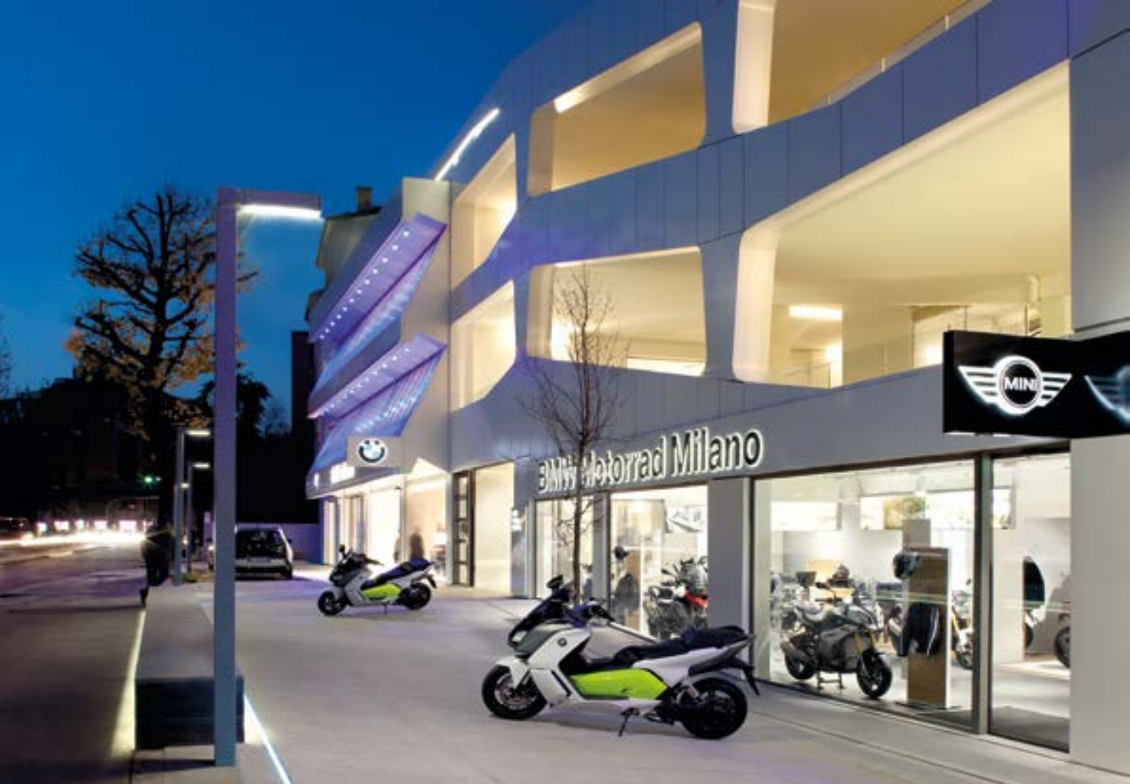
BMW Milan City Sales Outlet Via De Amicis, Milano, Italy / General contractor: ISG Italia © Ph. Barbara Corsico
